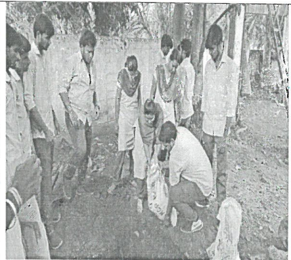
NSS Volunteer Students Digging Soak Pit
